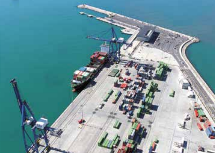
Port of Alicante Expansion. Alicante.
